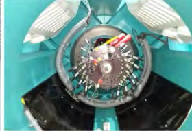
Camera Cable Wrap refrigeration fittings retrofit completed.
