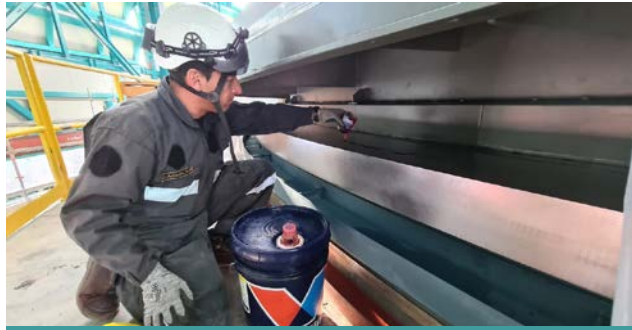
Keeping TMA azimuth bearing lubricated
