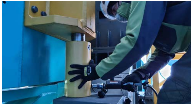
Maintaining TMA hydraulic jacks
