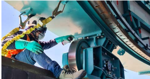
Lubricating the Dome bogies
